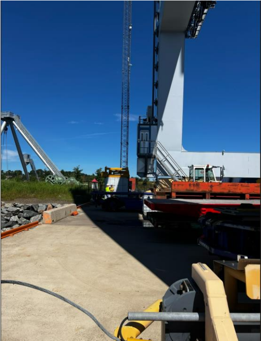
Location A (including the crane)
