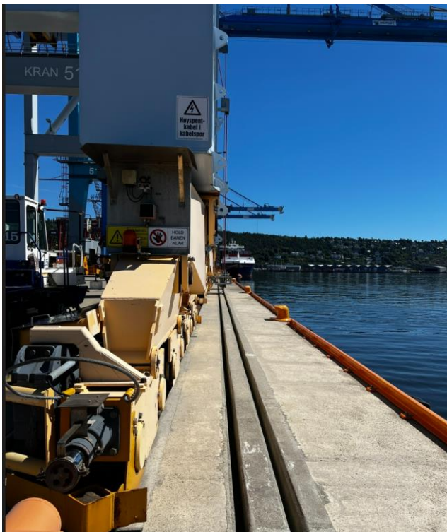
Crane rails, from location A
