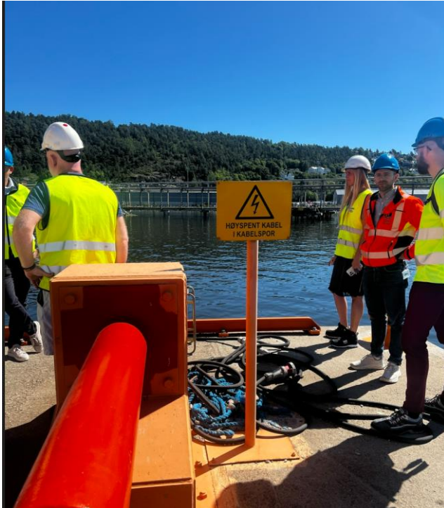
High voltage cable along the dock (both locations)
